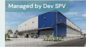
Matsudo Project Scheduled completion in Sep. 2024
