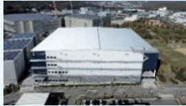
LOGIPOINT Kobe Nishi Completed in Nov. 2021
