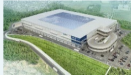
LOGIPOINT Fukuoka Kasuya Scheduled completion in Aug. 2024
