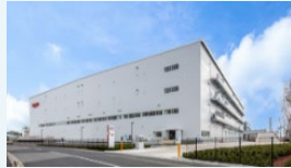
Matsudo Logistics Center Completed in Jan. 2022
