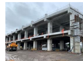
India High-Speed Railway Construction of Surat Station
