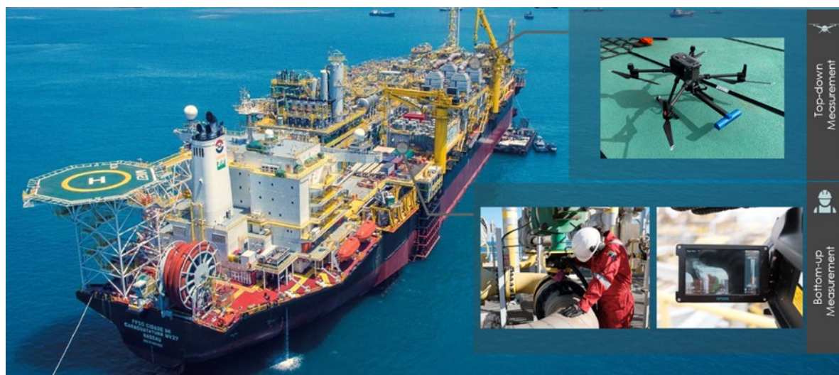
Figure 1: Measuring methane at an FPSO
