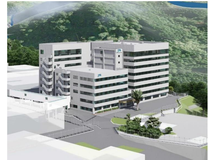
Construction to be Completed in May 2024
