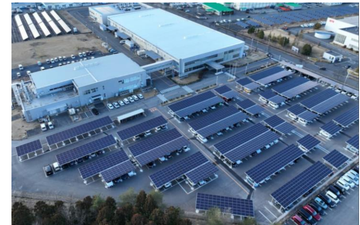
[Ichinoseki Plant (Iwate Prefecture)]
